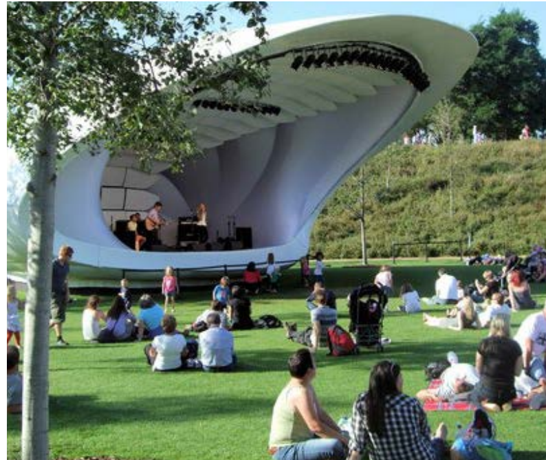
Sound Stage at Queen Elizabeth Olympic Park - London, UK
