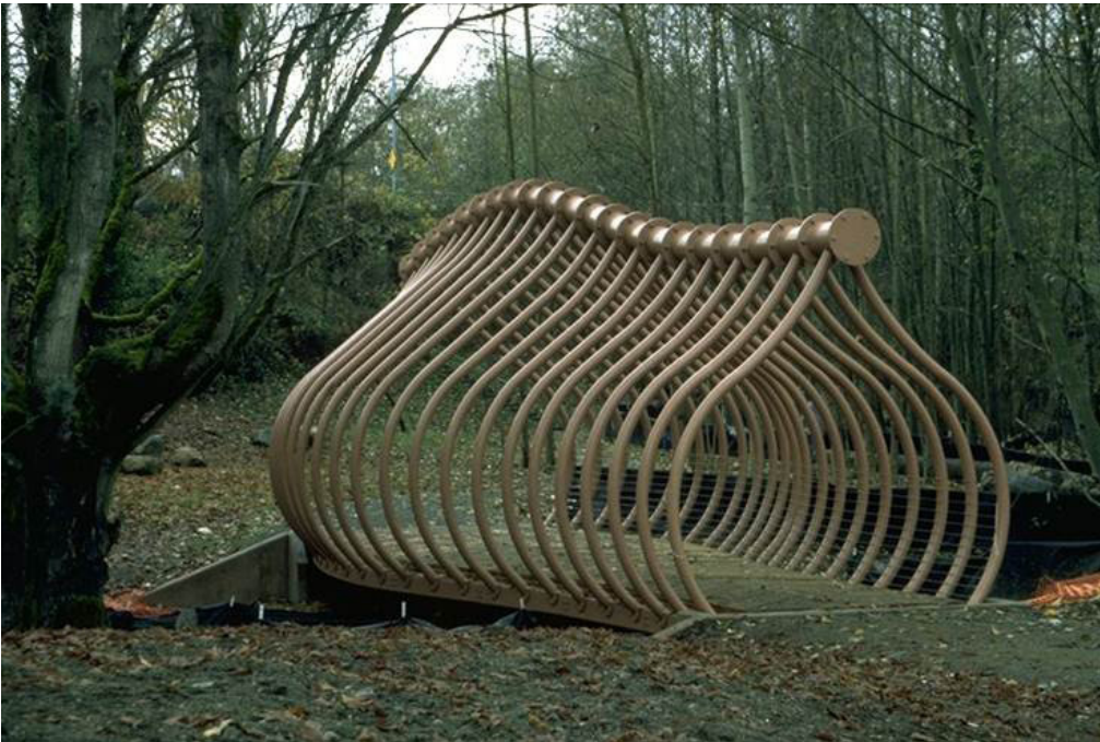
Fish Bridge, Longfellow Creek Restoration, Seattle, artist Lorna Jordan
