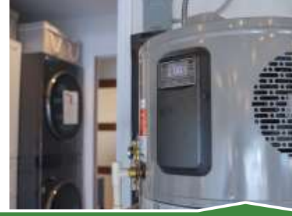
Emergency Water Heater Replacement
