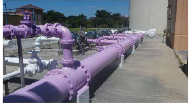
Purple pipe is used to designate reclaimed water and separate it from potable water. (Image Source: Brown and Caldwell)
