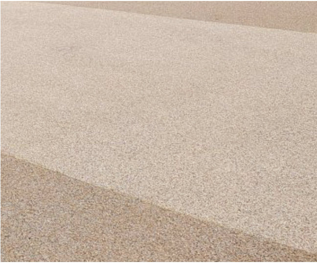
Custom CIP Concrete
