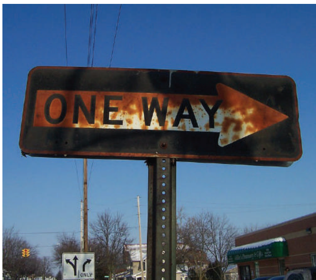
Signs that are not properly maintained
