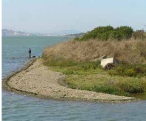
Erosion: Lagoon Beach
