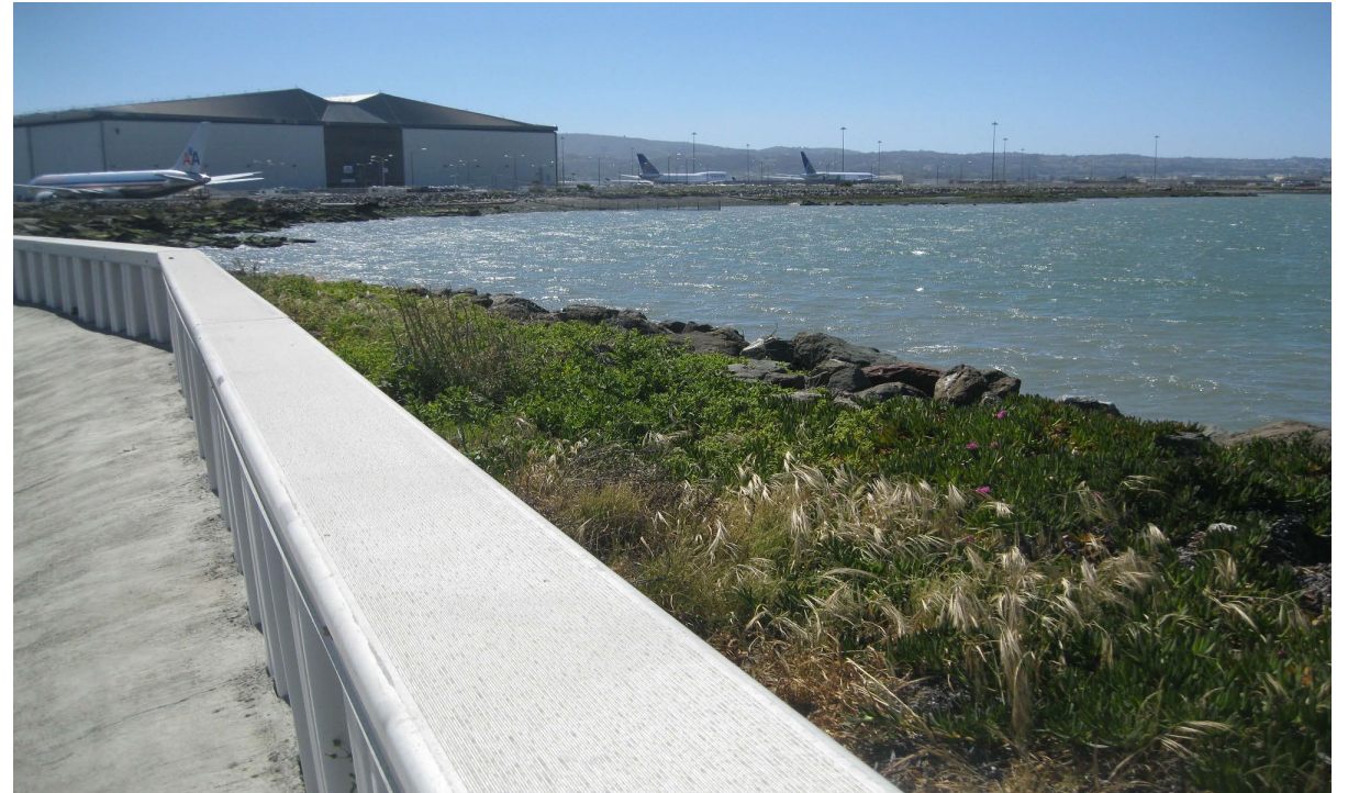
Vinyl Sheetpile at SFO
