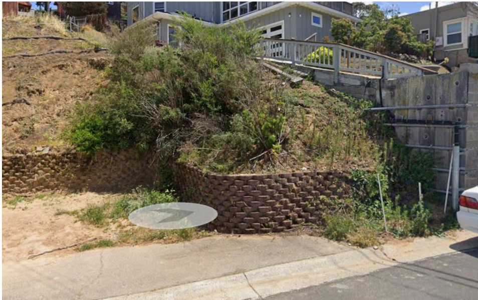
Santa Clara St. – bottom of stairway
